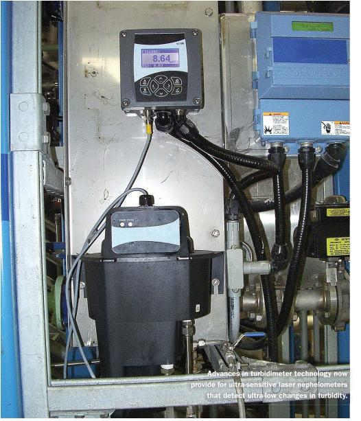
can't detect. However, long-term, successful application of laser nephelometers in membrane plants to detect small step changes in the filtering process indicates this instrument also can effectively monitor and optimize conventional granular media filter performance.
